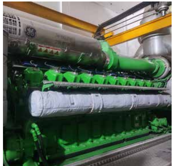
INNIO Jenbacher JMS 620 Type J gas engine at Suraj Cotton Mills Ltd, Raiwind, Punjab.
